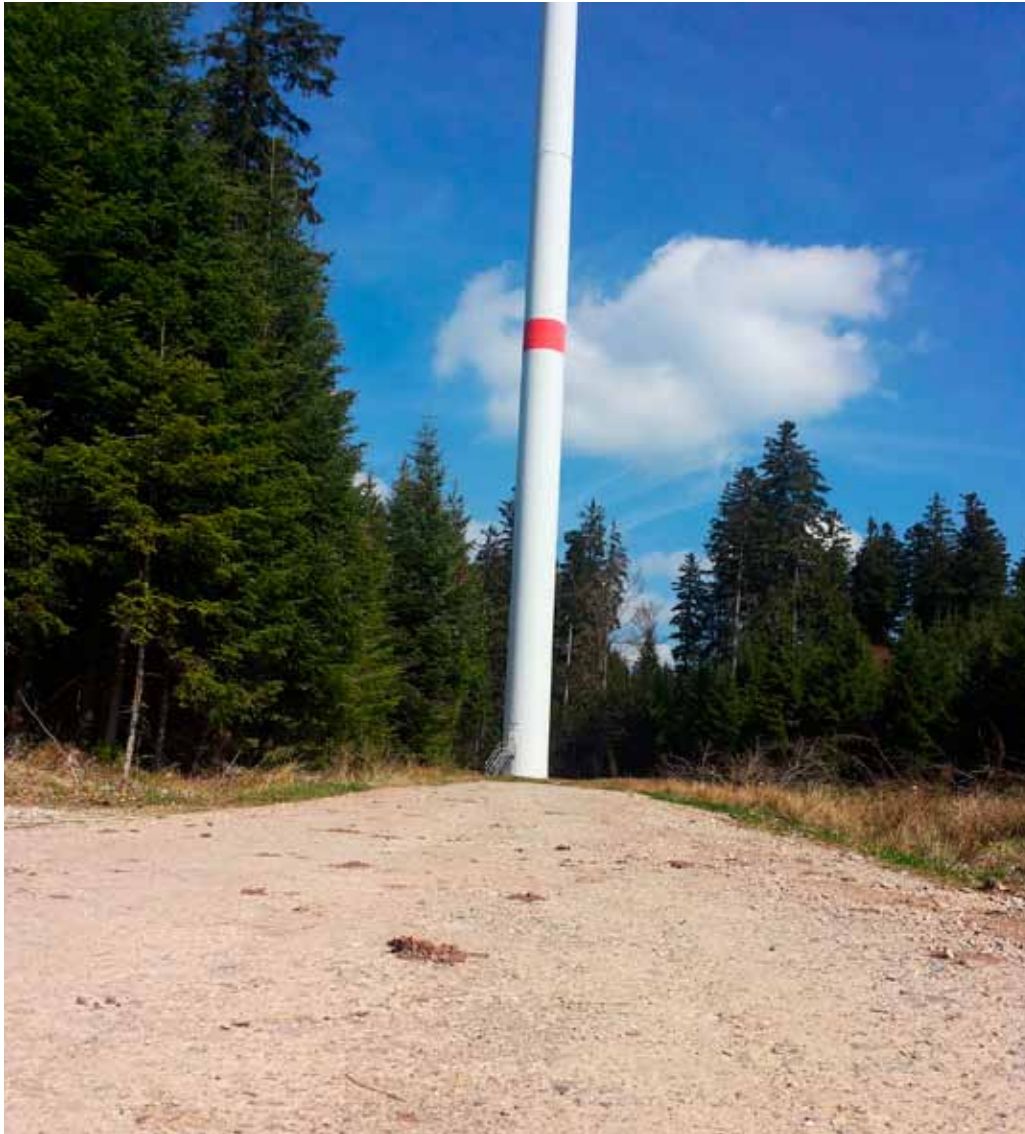
Status after more than 7 years (with heavy truck traffic and several strong frost periods)
